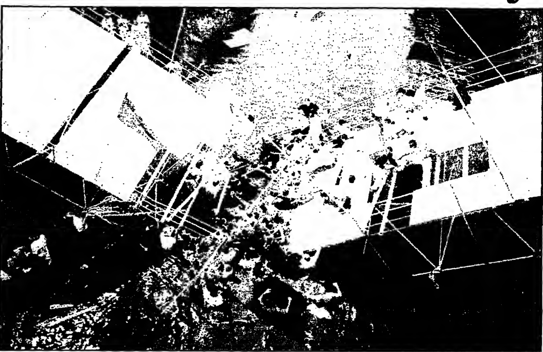
Rescuers evacuate victims from the collapsed footbridge over the Yarkon River last night.
